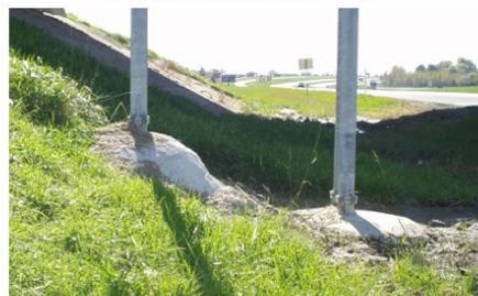
Concrete is poured above the level of the surrounding ground elevating the fixed portion of the breakaway device above the maximum 4" above the surrounding finished grade
