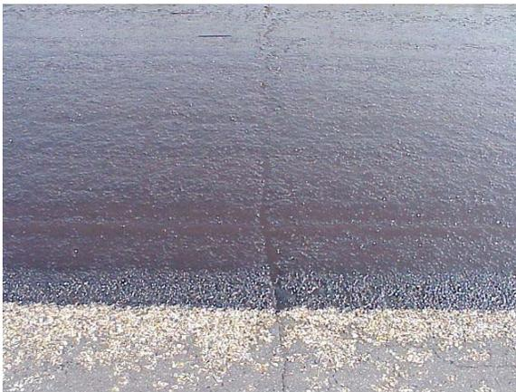
(3) Oil Penetrates and Seals Cracks
