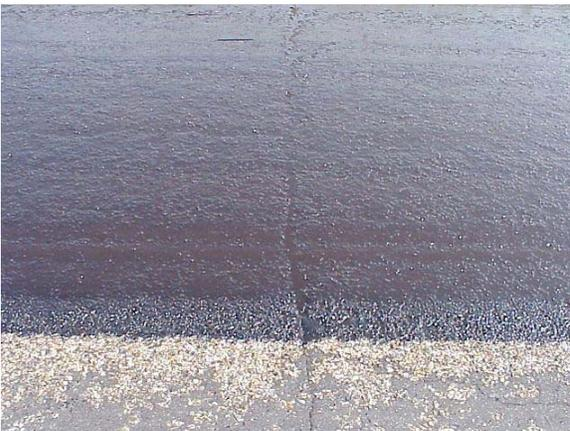
(3) Oil Penetrates and Seals Cracks
