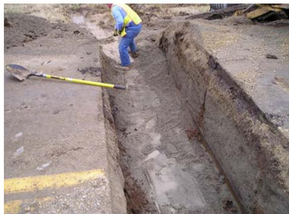
(4) Fine Grading Culvert Bed
