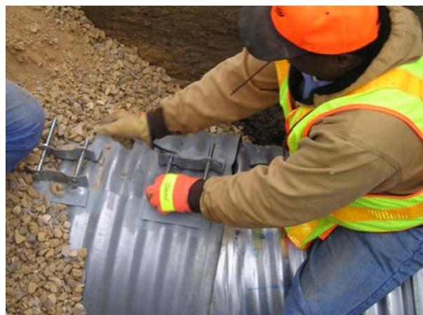
(6) Installing Pipe Connecting Band
