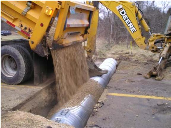
(7) Backfilling around Culvert Pipe
