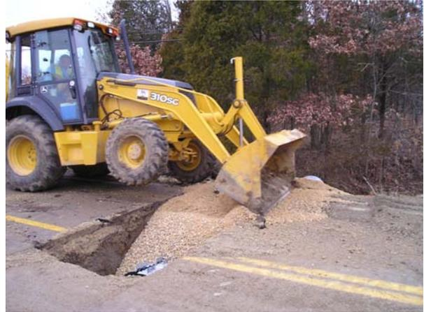
(8) Spreading and Compacting Pipe Fill
