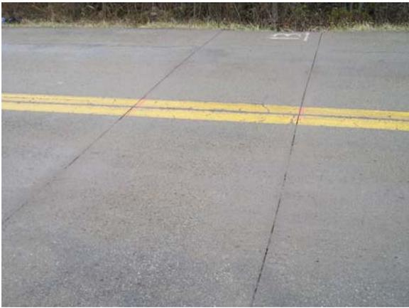
(1) Sawcut Pavement for Culvert Replacement
