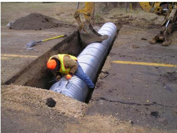
(5) Laying Culvert Pipe
