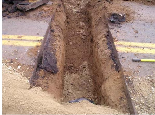
(2) Open Trench for Culvert Replacement
