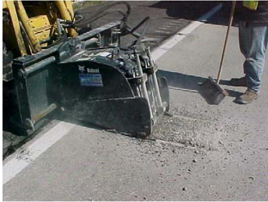
(8) Preping Pothole with Milling Attachment
