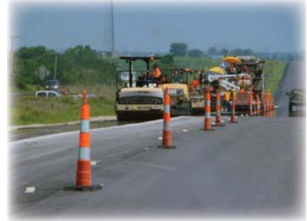
**Longitudinal buffer spaces** are to be used whenever practicable. Lateral buffer spaces may be considered based on the type of work.
