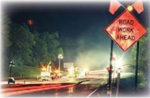
The first purpose is to illuminate a portion of the roadway in order to safely and effectively perform work activities or to highlight areas requiring increased driver attention. This is accomplished through work and area lighting, respectively. The second purpose is to supplement other temporary traffic control devices or to identify work vehicles and equipment. This is accomplished through warning and fleet lighting, respectively.
