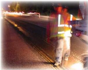
Typical work zone lighting may include dirigible lighting, portable light towers, balloon lighting, lights attached to equipment or post-mounted lights. In some cases, existing lighting or ambient lighting may meet lighting level requirements and negate the need for including work zone lighting.
