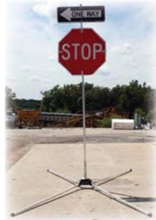
**Signs mounted in this manner may be left in place for up to three days.** An exception to this duration is any crosswalk/sidewalk closure, any road closure, Horizontal Arrow, Double-Headed Horizontal Arrow, Chevron, DETOUR (within arrow) or Gore Exit sign. These signs may be left in place for over three days.
