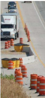
Any end of the barrier installation susceptible to being hit by vehicular traffic shall be protected with a crashworthy end treatment. This requires installation of a barrier height transition for speeds less than or equal to 35 mph or an approved crash cushion for speeds greater than or equal to 40 mph. As an option, the barrier may be flared at a rate of 8:1 back to the limits of the clear zone, back slope or curb provided the side slope is 1V:6H (6:1) or flatter.
