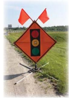
**Mounting heights for regulatory and guide signs are as specified for post-mounted signs.** Portable signs may be located adjacent to or within the roadway itself. **However, a minimum lateral clearance of three ft.**, measured horizontally from the edge of the sign to the edge of the designated traveled way, is recommended.
