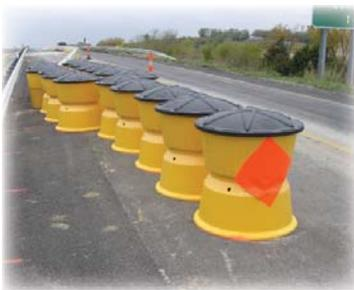
Crash cushions mitigate the effects of errant vehicles impacting roadside obstacles such as fixed objects or exposed barrier and guardrail ends. The system is designed to accomplish this by either smoothly decelerating the vehicle to a stop or redirecting the vehicle.
