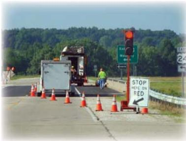
Temporary traffic control signals are used at haul road or equipment crossings, on one-lane, two-way operations, and at temporary intersections located within the temporary traffic control zone to assign vehicular right of way. Typically, this is done with temporary span-wire installations or trailer-mounted units.
