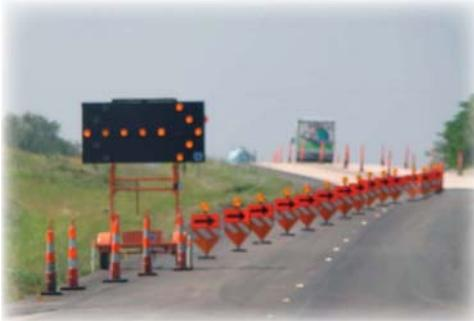
Temporary traffic control devices are the medium through which traffic is informed of and guided through a temporary traffic control zone or otherwise protected from an unsafe condition. The most common devices include signs, portable changeable message signs, flashing arrow panels, channelizers, barricades, temporary traffic barriers, pavement markings, lighting devices, temporary traffic signals, crash cushions, protective vehicles and truck-mounted attenuators.
