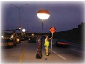
**Warning lights** are an option available to increase the target value of other temporary traffic control devices. Typically, a single self-contained unit that emits a yellow light is used for this type of lighting.
