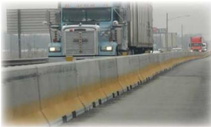
Due to the amount of resources needed to put barrier in place, this option is generally reserved for long-term stationary operations where the need for the noted function is critical.
