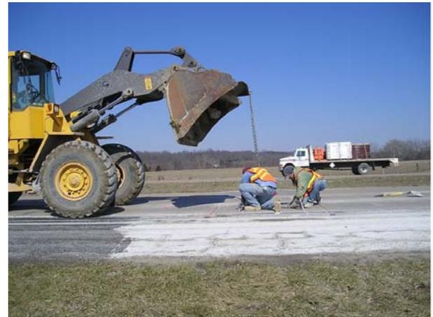
(4) Concrete Slab Removal Set Up
