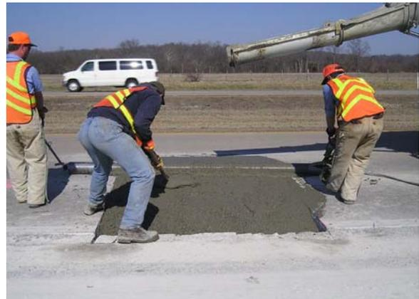
(10) Machine Finish Concrete with Bunion Tube
