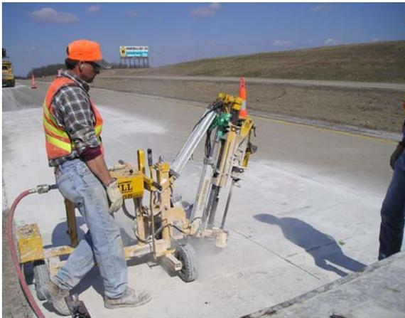
(3) Concrete Slab Replacement Drill Prep
