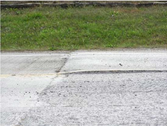
(3) A Completed Milled Pavement Joint
