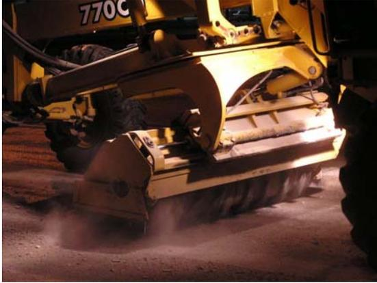
(1) Roto Grader Milling a Pavement Joint
