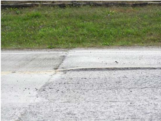
(3) A Completed Milled Pavement Joint
