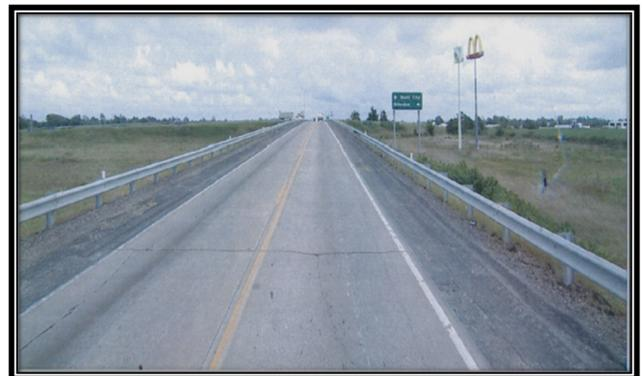
A preventative maintenance treatment might be used on this #6 ranked pavement to keep the roadway in good condition.
