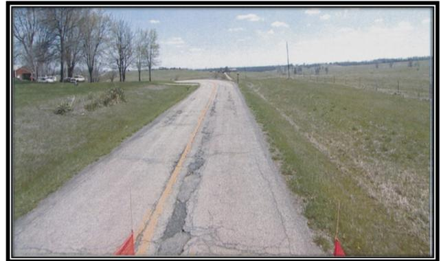
On the 1 to 10 Pavement Rating Scale, a more substantial treatment than what would be used on a higher ranking pavement may be required to get this #3 rated pavement in good condition.
