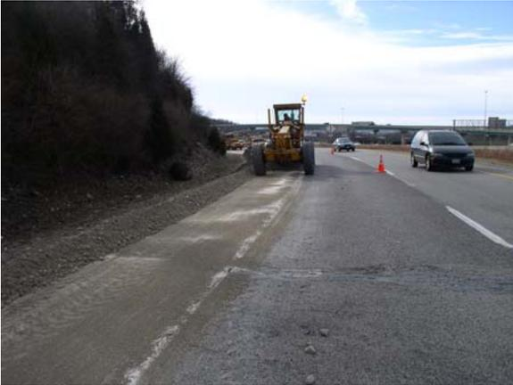
(15) Blading 2" Aggregate with Motograder
