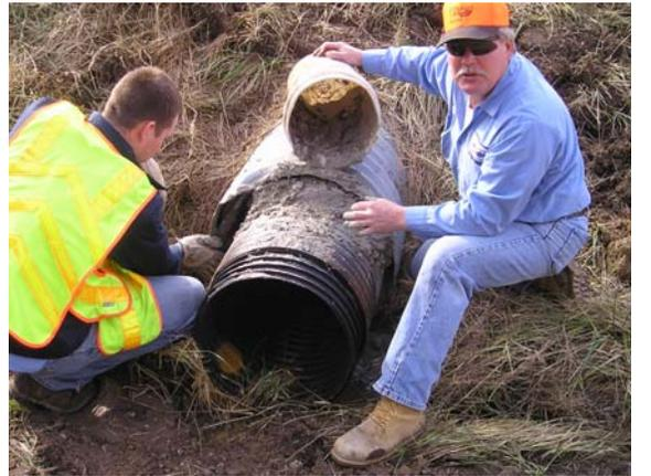
(10) Grouting Pipe Liner to Culvert End
