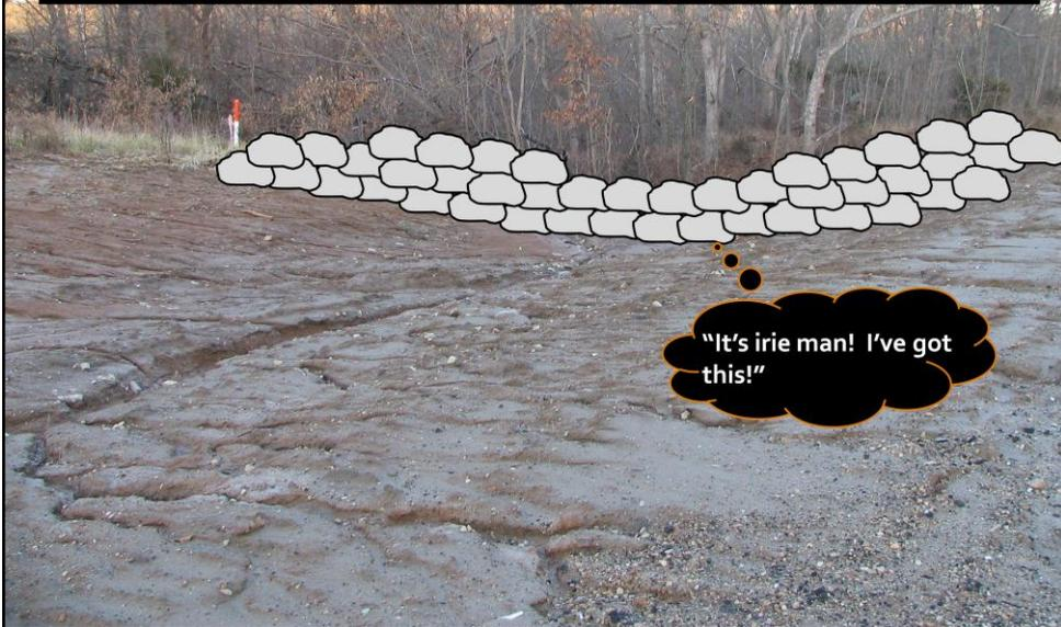
**Silt fence is NOT an “appropriate impediment” to sediment movement at an outfall location. An outfall location such as this must be identified on the site plan. Site plans with “silt fence” shown at the “outfall location” should raise a red flag to anyone who reads the plans (site map). Install robust devices at outfall locations.**
