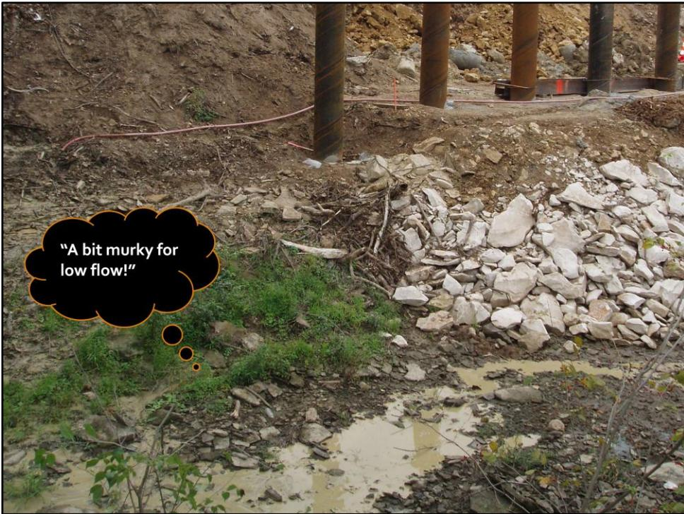
**This dewatering operation is pumping turbid, brown, contaminated water from a drilled shaft directly into a clear stream. Clearly pollution because the stream is clear as it flows into the job.**
