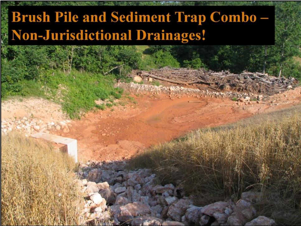
**Brush piles can help impound and filter stormwater. Following installation make certain that the structure is “tight” enough together and to the ground to impound water and sediment.**
