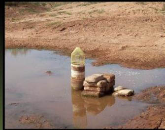
When using flocculants surface skimmers should definitely be considered to draw clean water from the top of the water column.
