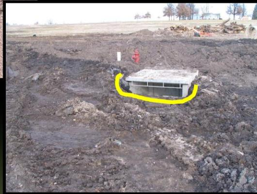
**Carefully evaluate all inlet protection for desired performance, safety and potential ponding/flooding concerns.**
