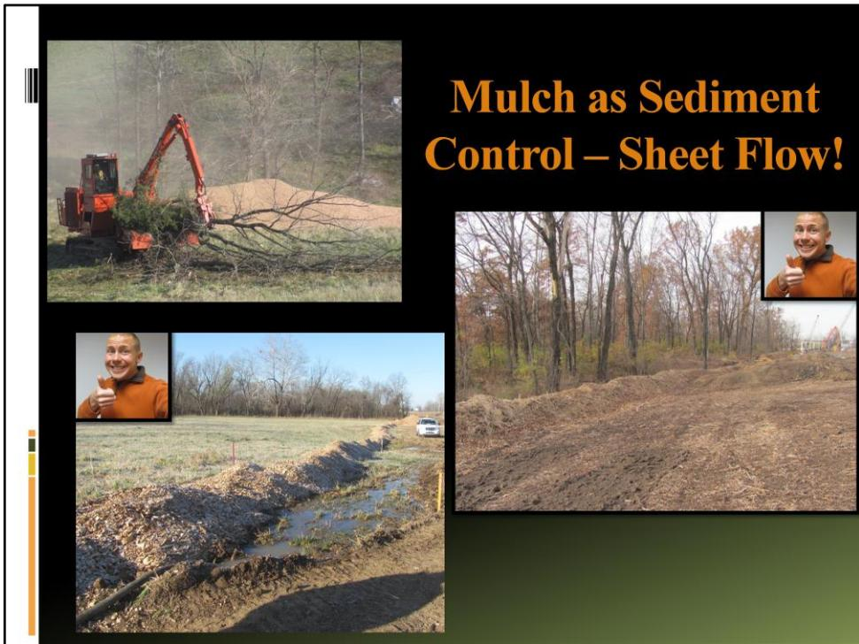
**Wood mulch produced on the job can be used for erosion control or sediment control. The MoDOT SWPPP allows for the use of perimeter mulch berms as a “silt fence” application.**
