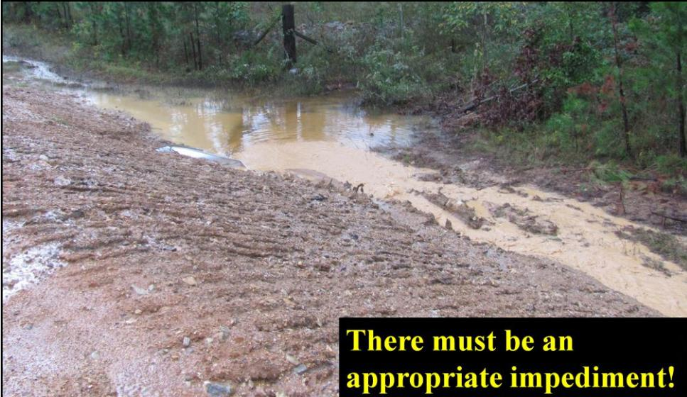
**No outfall controls...no slope stabilization....disaster!**
