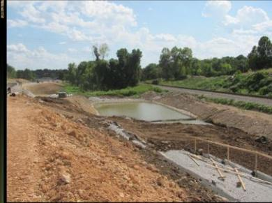
**Always install outfall and perimeter protection prior to grading.**
