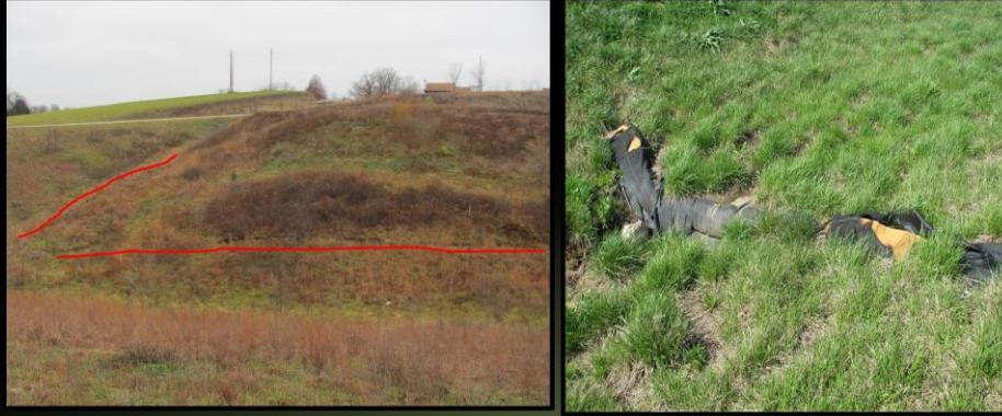
**Don't remove your BMPs until you are comfortable that the area is no longer susceptible to erosion. But they must be removed if they are not biodegradable!**
