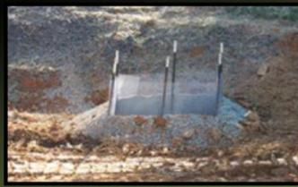
This is an introduction to this device that was added to the MoDOT SWPPP. It will stand up to heavy flows and filter stormwater with the small stone, which makes it a good perimeter or inlet protection BMP.
