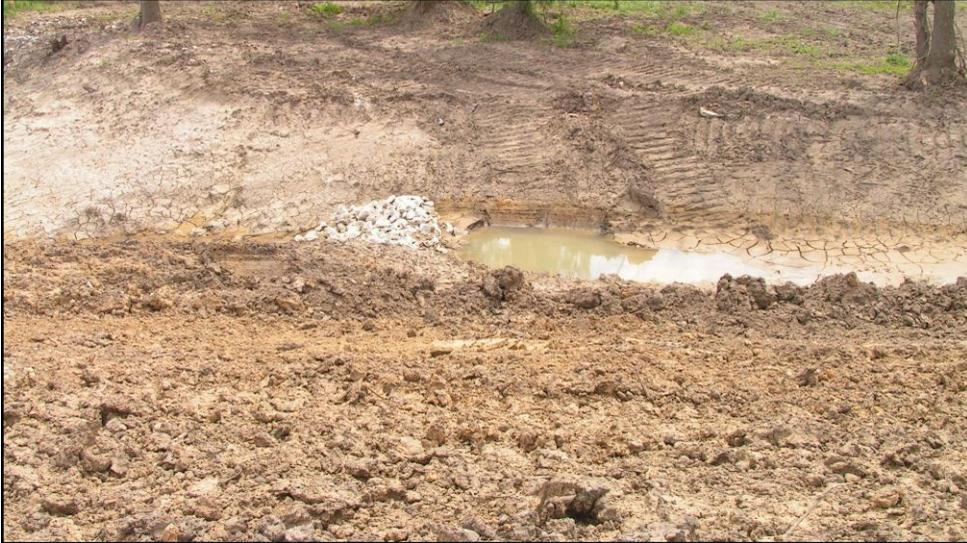
Surface roughening is a very temporary BMP. Do not try to use surface roughening as a stand alone BMP for extended periods of time.
