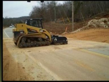
The most commonly used is a rocked construction entrance, but it takes a lot of maintenance to keep it functional under heavy traffic.
