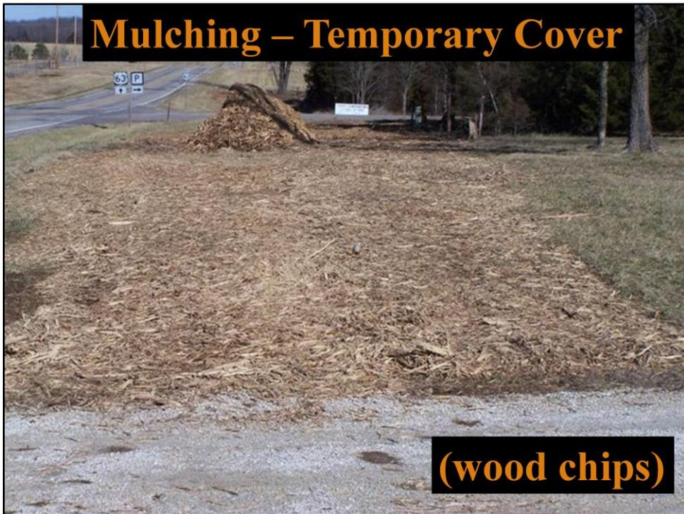
**Bark mulch, in combination with downgrade ditch check, sediment trap, sediment basin or silt fence is considered interim stabilization. Be careful with fresh mulch on a job, as it can affect soil pH as it breaks down.**
