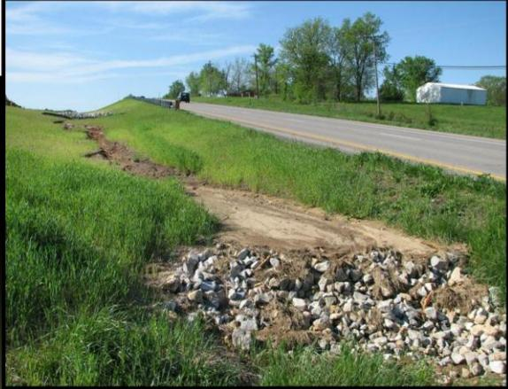
Always try your best to space ditch checks “toe to top” down your ditch grade (the top of the down grade check should be equal in elevation to the toe of the one immediately upgrade from it as shown in Figure 5.2). This will prevent scour and erosion within your ditch line and help limit the likelihood of overwhelming the downgrade checks with sediment.
