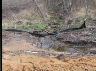
Typically staked geotextile is synonymous with silt fence, but there are other devices that can meet the silt fence requirement. Understand the difference between perimeter controls and ditch controls.
