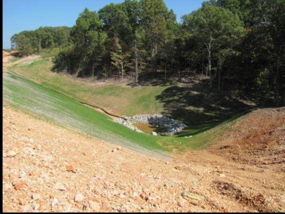
**If you can, include inlet protection at the temporary slope drain inlet as well – *treat sediment as close to the source as possible***
