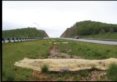
**YOU WILL NEED TO UTILIZE DITCH CHECKS ON YOUR PROJECTS!!** Ditch checks are probably the most commonly used BMP at MoDOT since we have so many water conveyance channels on our right of way.
