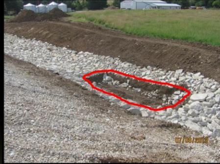
Sediment traps are very common outfall devices on MoDOT projects due to right of way constraints.
