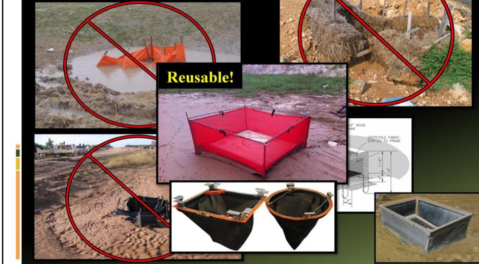
Inlets are places of concentrated flow and should never have “silt fence” type devices installed around them that utilize non-reinforced frames, such as these staked geotextiles and straw bales.
