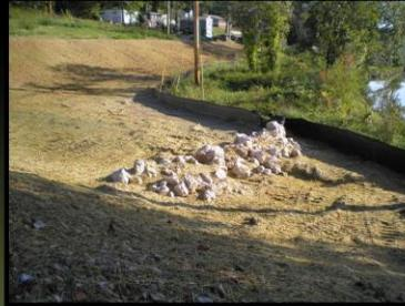
**GEOTEXTILE SILT FENCE MUST BE KEYED INTO THE GROUND AT LEAST 6 INCHES AND HAVE A FLAP OF APPROXIMATELY 4 - 6 INCHES POINTED TOWARD THE UPGRADE SLOPE!!!! If you don't do this, it will likely undermine in short time!**
