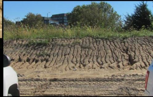
Be sure the last pass runs the equipment up and down the slopes vertically, leaving horizontal depressions!
