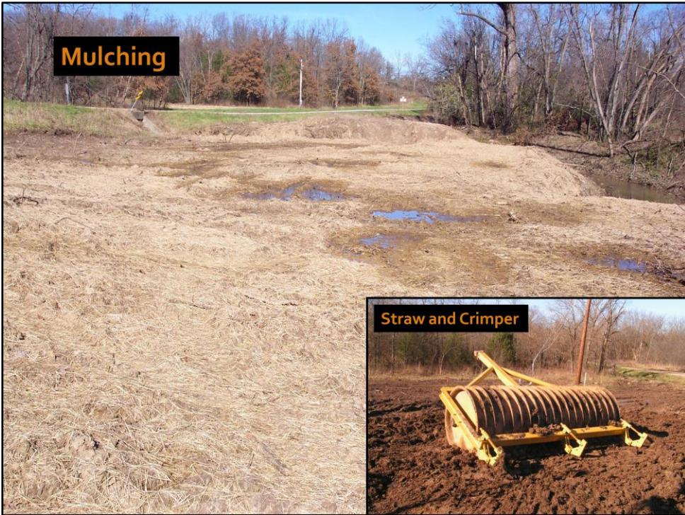
**Crimped or tacked straw is considered interim stabilization when used in conjunction with sediment control devices.**
