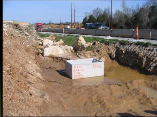
“Riser pipe” is described in SWPPP in the section on Inlet Controls. Clean out will be necessary.
